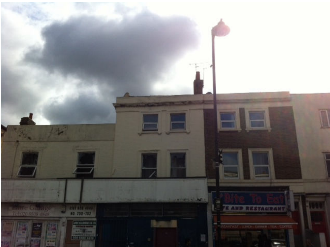
Existing Tottenham High Road Frontage
